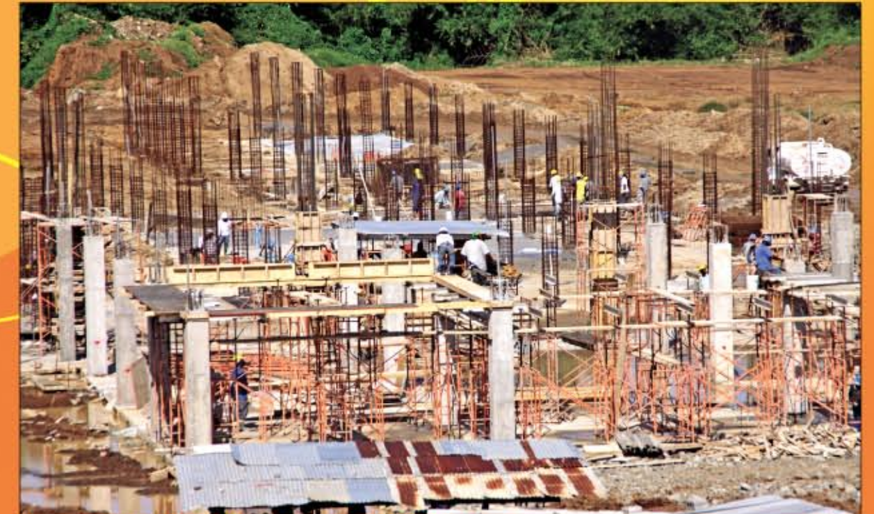
Men hard at work on the terminal building
