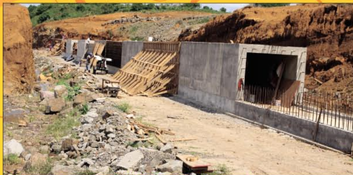
Culverts under construction in the 2nd kilometre
