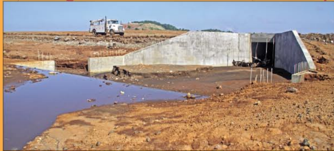
The water intake for the box culvert in the 1st kilometer
